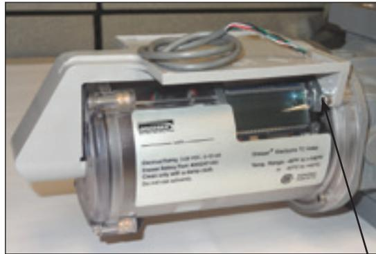
Figure 8.59-Insert the 7/8-inch (long) screws
